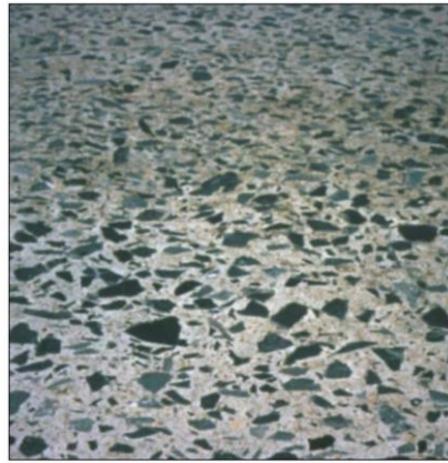
Gambar 9.16. Polished aggregate pada perkerasan kaku (Sumber : U.S. Department of Transportation, 2014)
