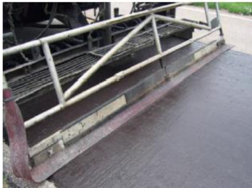
Gambar 11.4. Implementasi Micro surfacing
