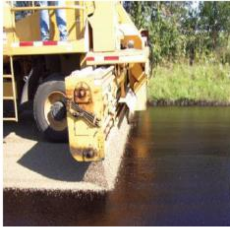
Gambar 11.3. Implementasi chip seal
