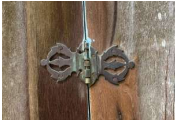
Gambar 2. 35 Detail Engsel Jendela Sumber: Tim Kontributor, 2024
