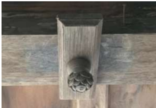
Gambar 2. 34 Detail Detachable Window Lock Sumber: Tim Kontributor, 2024
